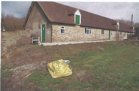
The barn roof for rainwater
